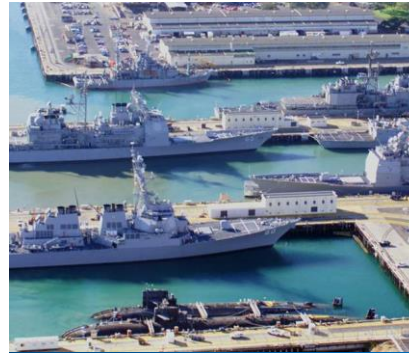
Pier 5 Replacement, VA
