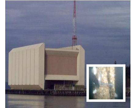
Explosive Handling Wharf, Bangor WA
